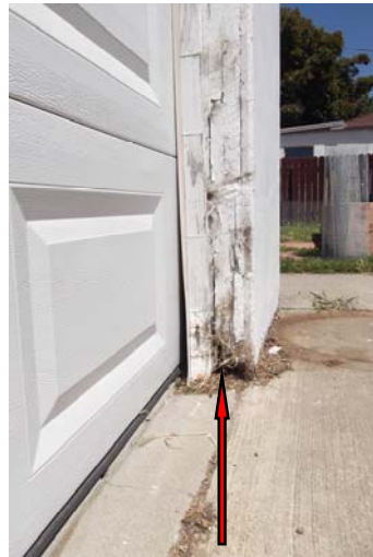
Trim Deterioration
