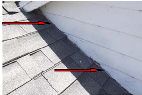
Missing Flashing
