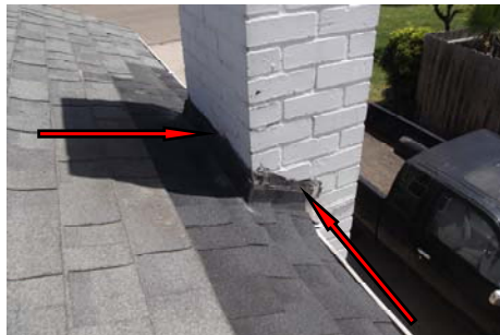
Improper Flashing
