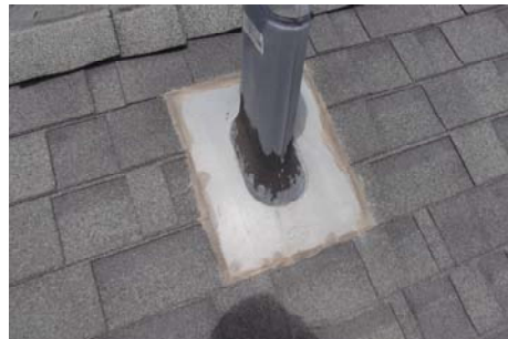
Improper Flashing
